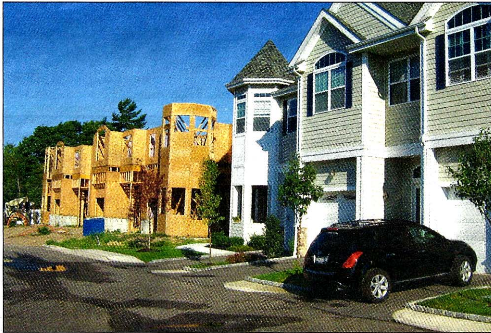
Finished townhouse sits next to hollow building frames at Riverview on the Patchogue River.
